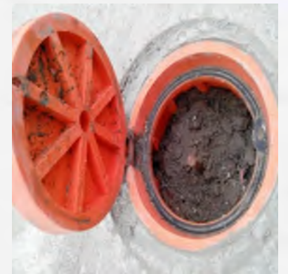
Ground Settlement Marker
