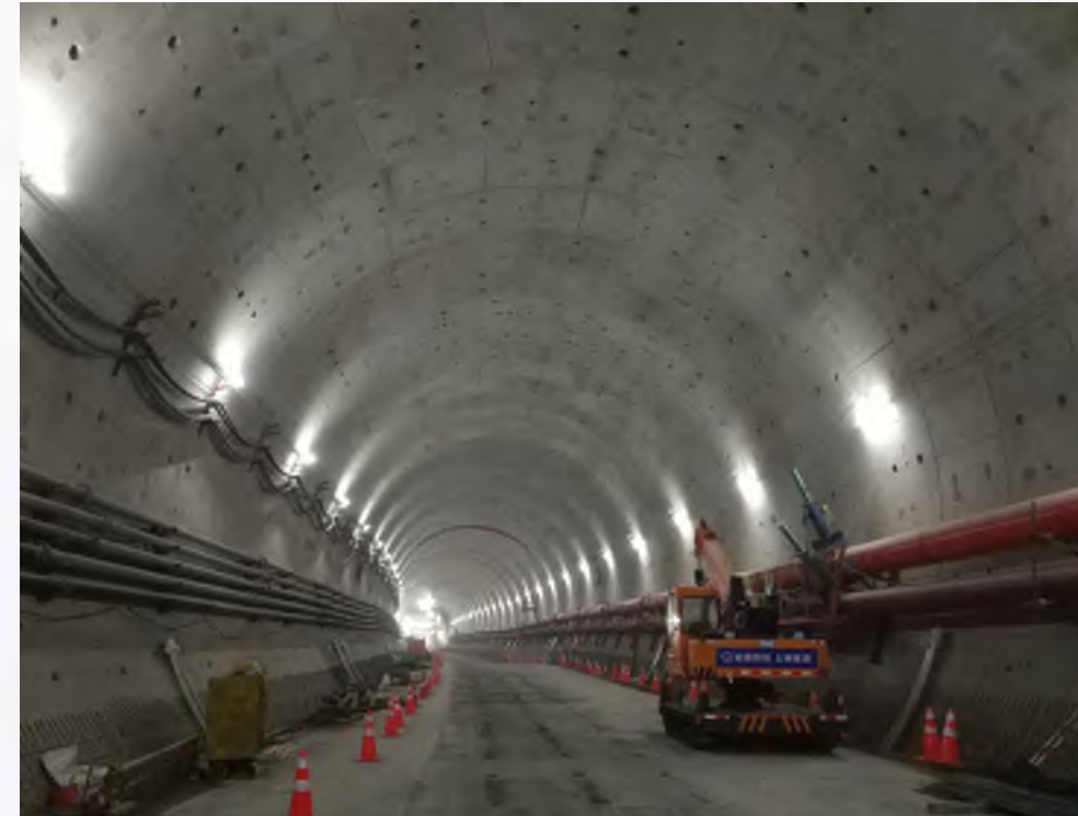
First Drive Completed
