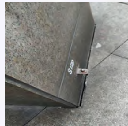
Building Settlement Marker
